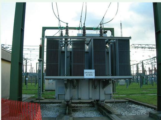
**Figure TF26-1:** A large 50 MVAR (Mega-Volts-Amps Reactive) loading inductor.
