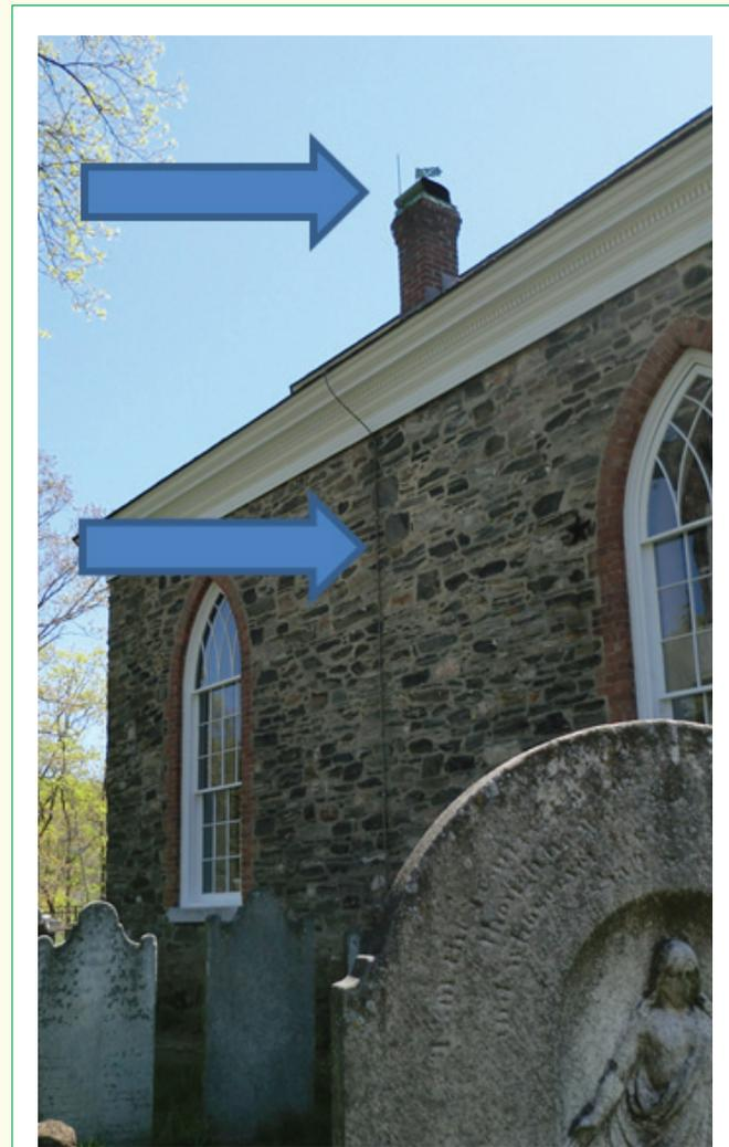
**Figure TF2-2:** Lightning rod and grounding cable on Old Rock Church at Sleepy Hollow, New York. The lightning rod attracts the strike by concentrating charges at its tip. The cable shunts the current to ground, carrying it on the outside of the (rock) church, rather than on the inside where materials (wood, plaster, etc.) are more flammable. The cable is large enough in diameter to carry the current without burning, although it will still be hot to the touch after a lightning strike.
